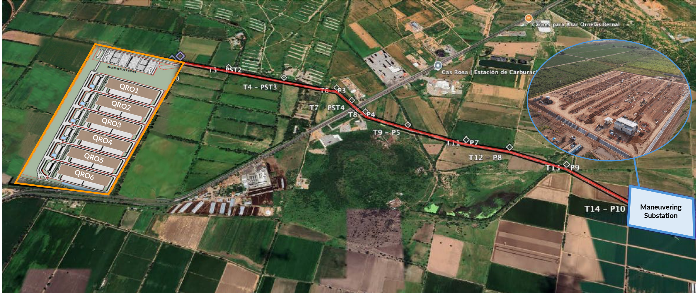
— CHQ QRO Campus — Maneuvering Substation
